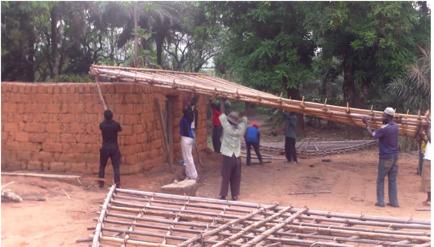
Figure 51: Lifting the roofs on to the house top
