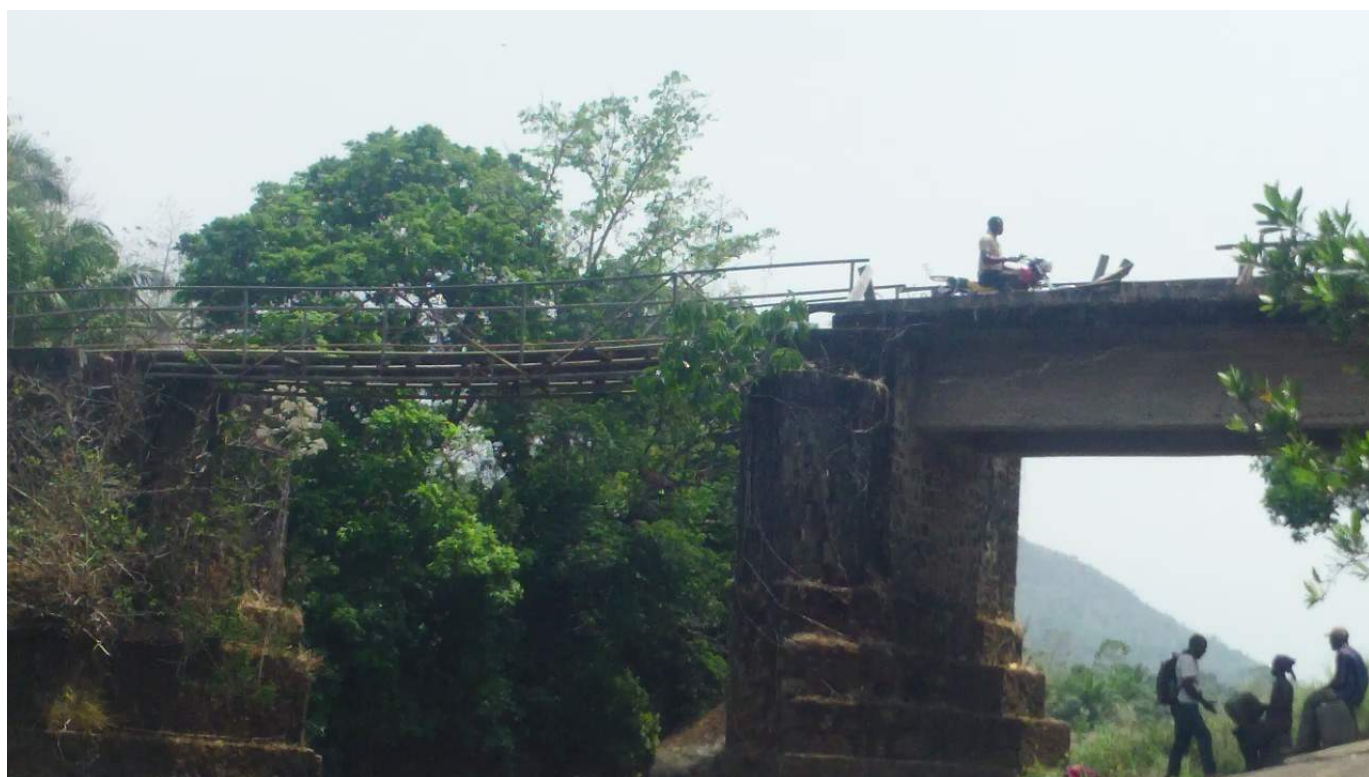
Figure 43: Crossing river: Mbuk(right) from Fonfuka (left)
