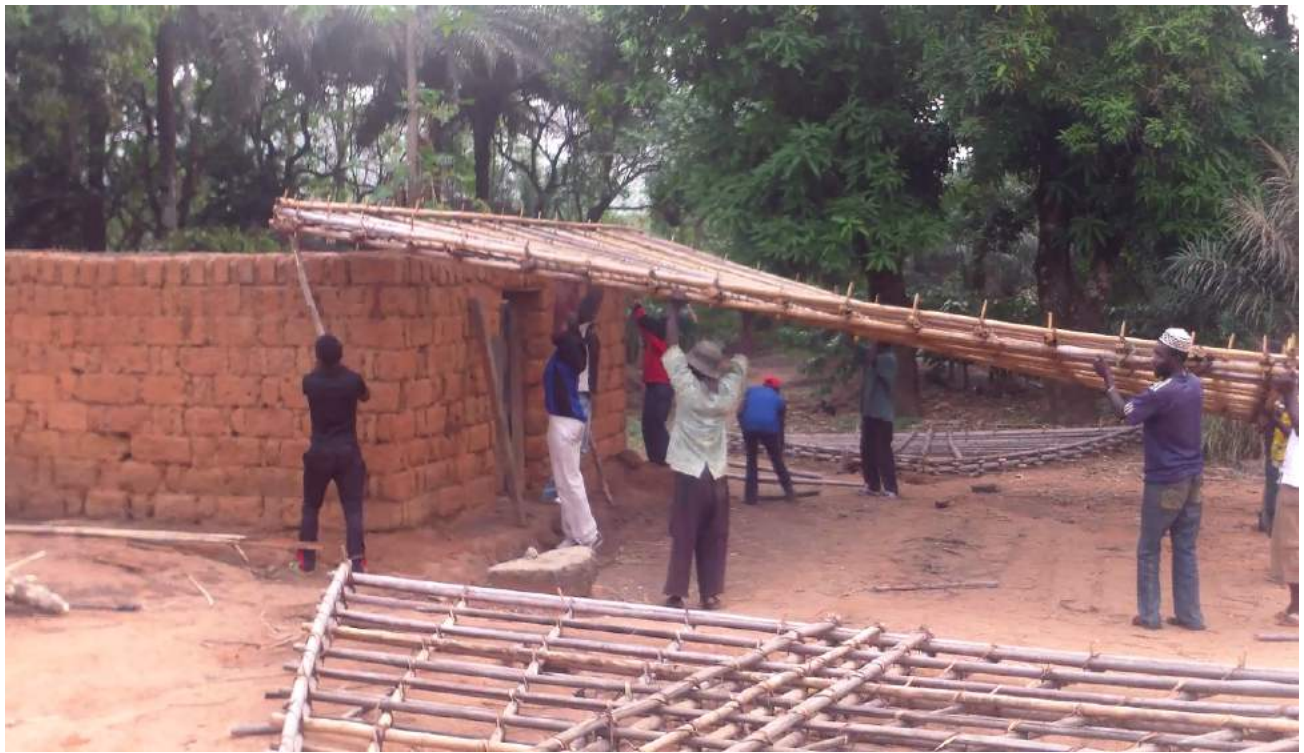
Roof from the ground carried onto the house top (in Aghem, it is constructed on the house top)
