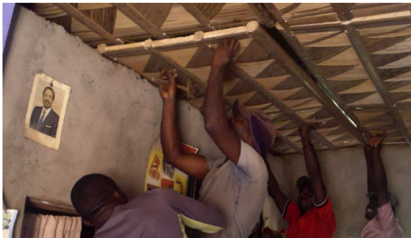
Arts & craft, Fitting the ceiling at the Mbuk palace, 31 st December 2014
