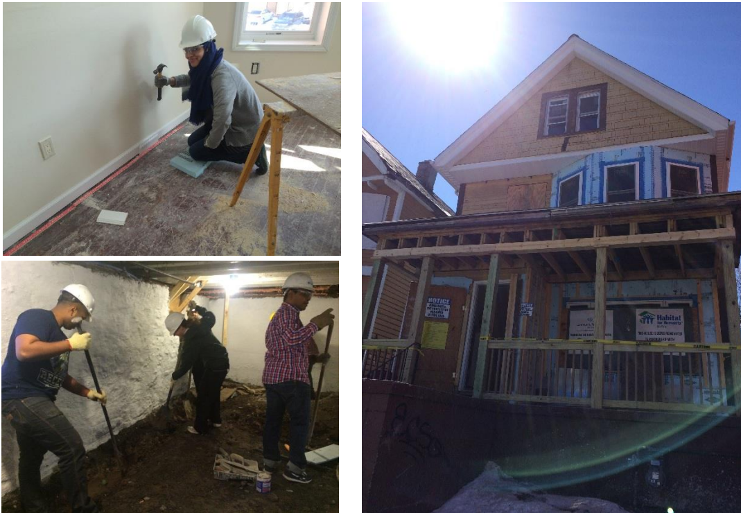
Graduate students helping with the renovation of the house
