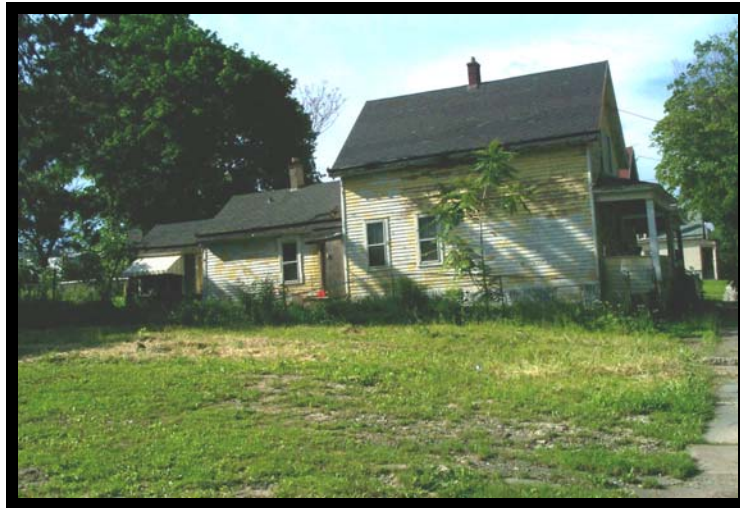
Figure 2: Dilapidated Housing in the Fruit Belt
