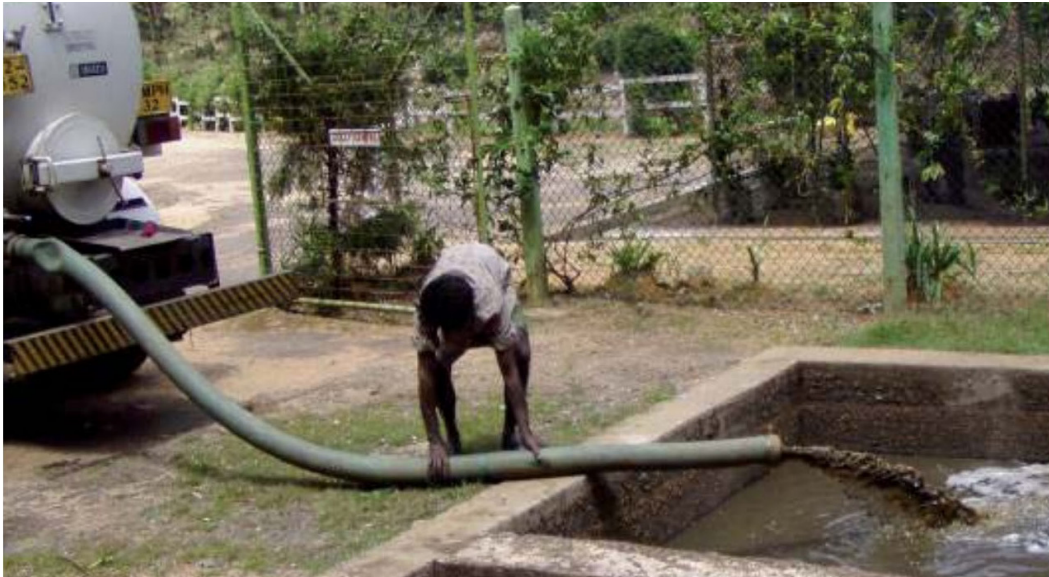
Figure 18: Lime stabilization pit
